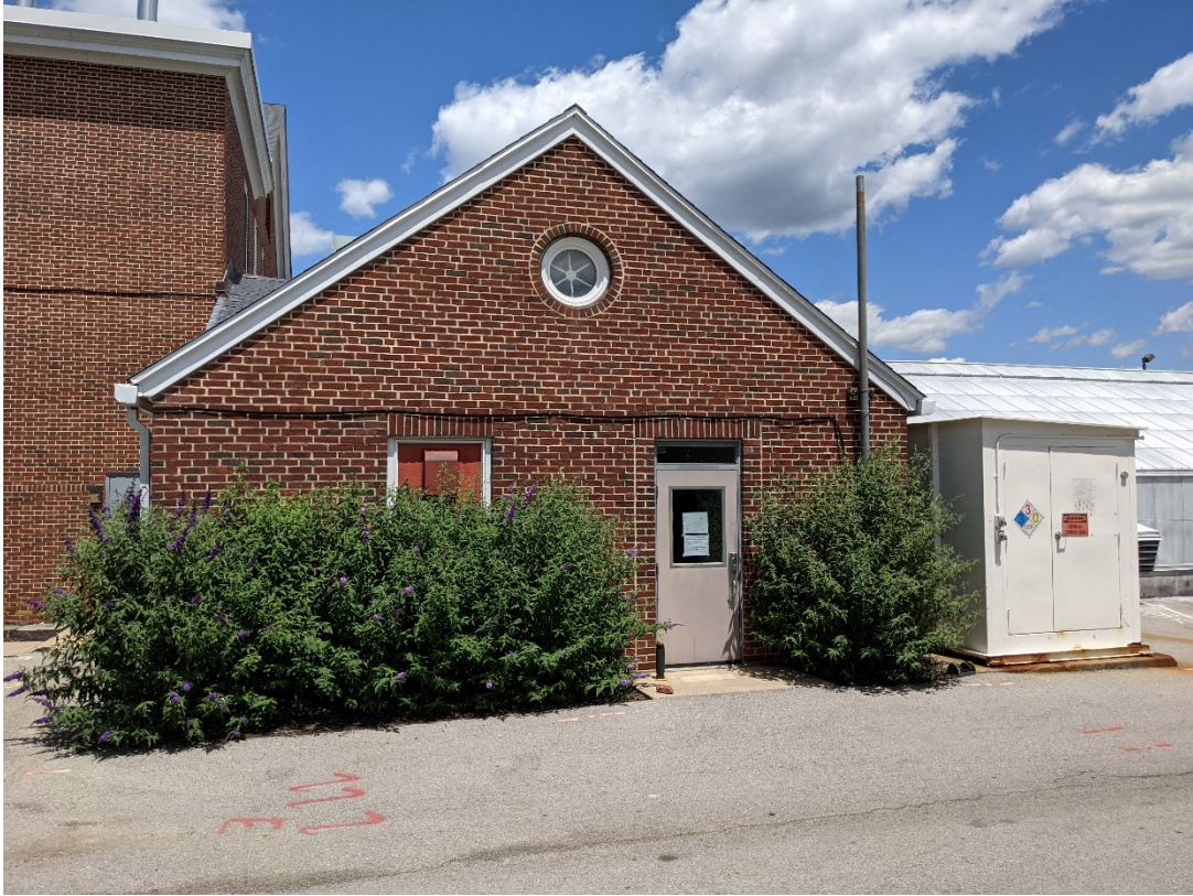
Figure 3: Bldg 005 (headhouse), photographer facing northeast
