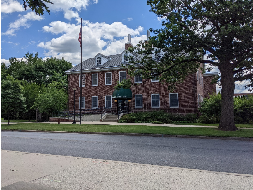
Figure 1: Bldg 004 (laboratory/office), photographer facing southeast
