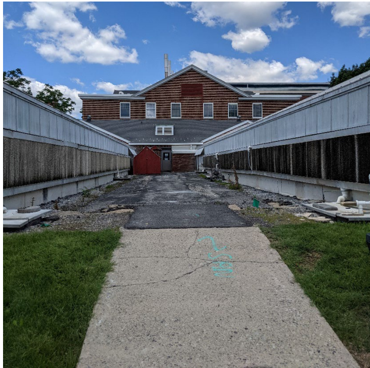
Figure 4: Bldgs 001 (greenhouse), 002 (greenhouse), 005 (headhouse), and 004 (laboratory/office), photographer facing northwest
