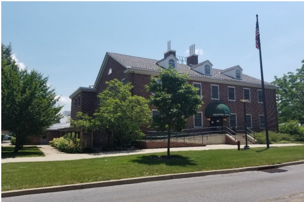
Figure 2-1: Buildings 004 and 005; Photographer facing southeast
