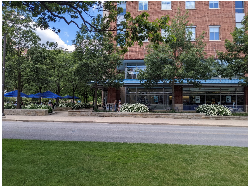
Figure 8: View from sidewalk in front of Bldg 004 (laboratory/office), photographer facing northwest
