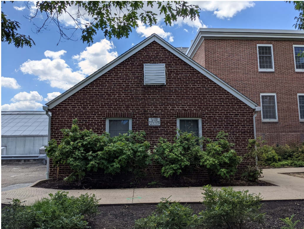
Figure 5: Bldg 005 (headhouse), photographer facing southwest
