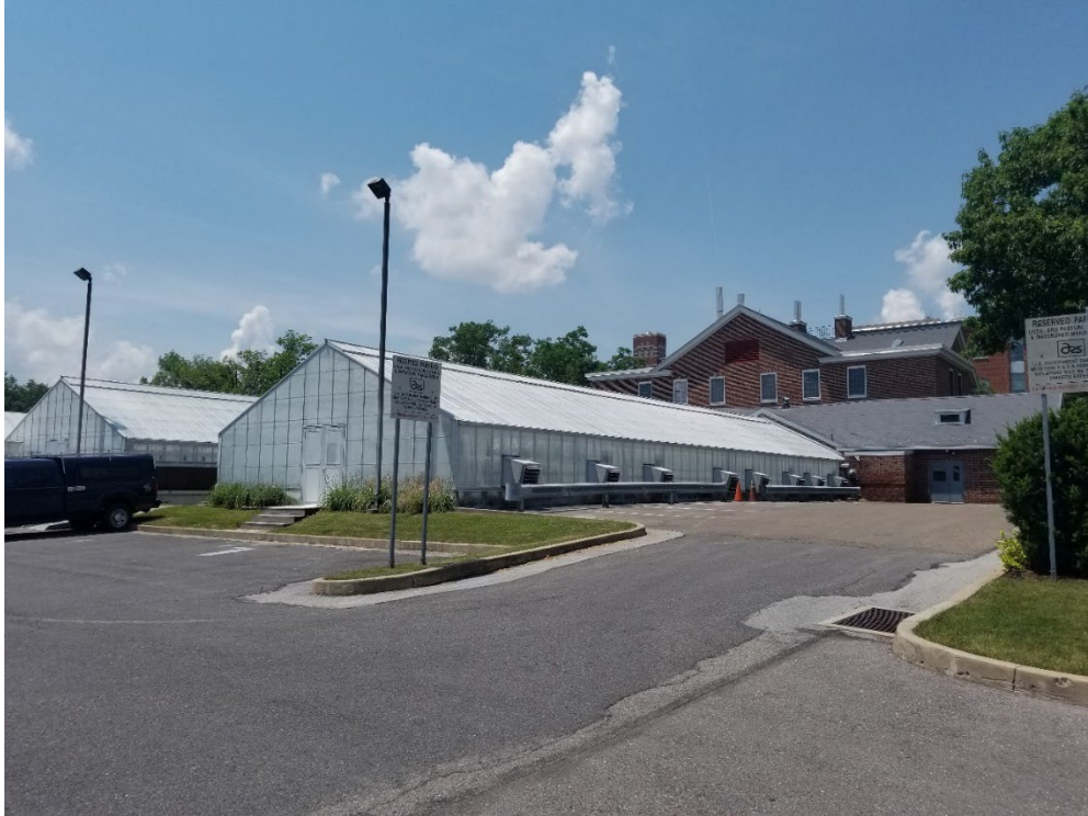
Figure 2-2: Buildings 001 and 002; Photographer facing northeast
